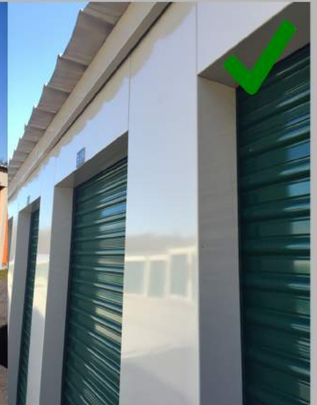
HALEY METAL BUILDING SYSTEM AFTER 5 YEARS
